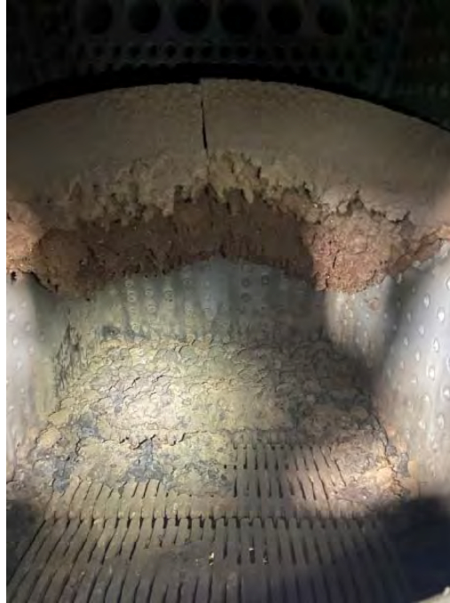
Front half after dropping back half
