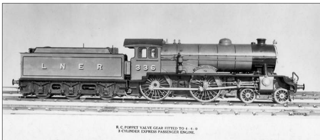
Figure 14 LNER Shire RC Poppet valve gear
